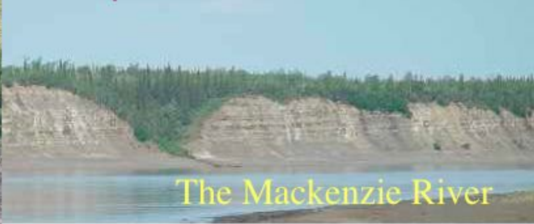
Examples of river bank erosion
